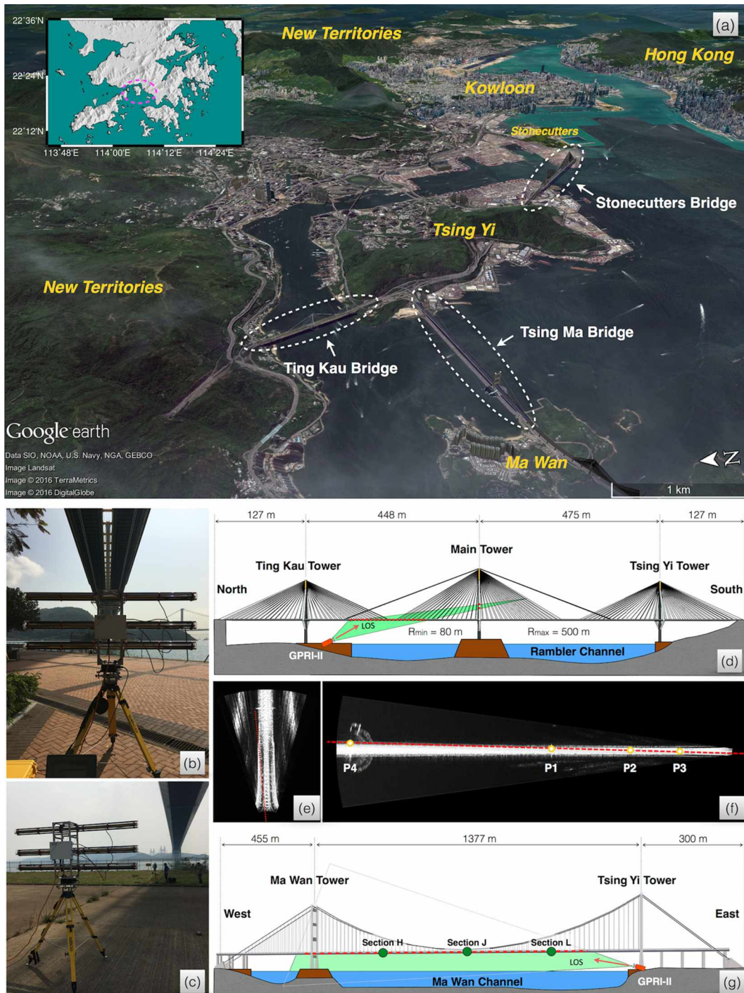
Fig. 4. (a) Locations of the two bridges studied. (b) The GPRI set up under the Ting Kau side of the TKB. (c) GPRI set up below the Tsing Yi Tower. (d) Measurement geometry for TKB. (e) Radar intensity image from TKB. (f) Radar intensity image from TMB, where P1, P2, P3, and P4 are the locations of one-half, one-quarter, and one-eighth of the mid-span, and the Ma Wan Tower, respectively. (g) Measurement geometry for TMB, where L, J and H are the locations of GPS stations. Red lines in (e) and (f) show the imaging direction of the FAS monitoring. (For interpretation of the references to color in this figure legend, the reader is referred to the web version of this article.)
