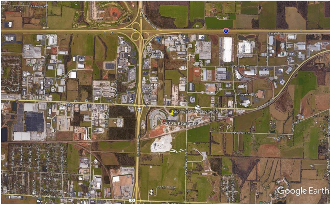
Figure 5.1. Google Earth map showing the location of Springfield Underground.
