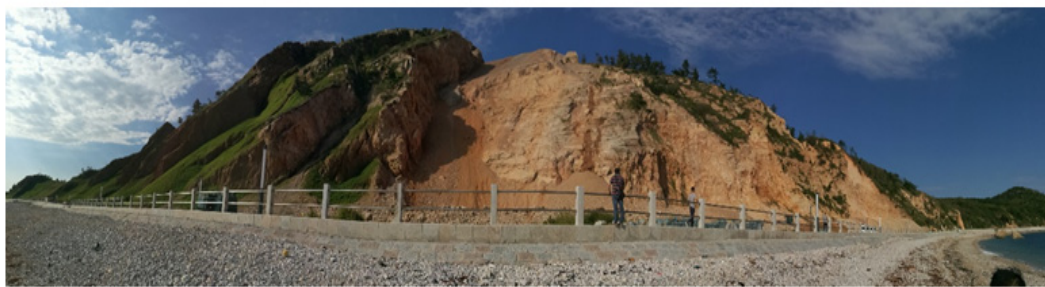
Figure 2. Landslide scene of Beichangshan Island.
