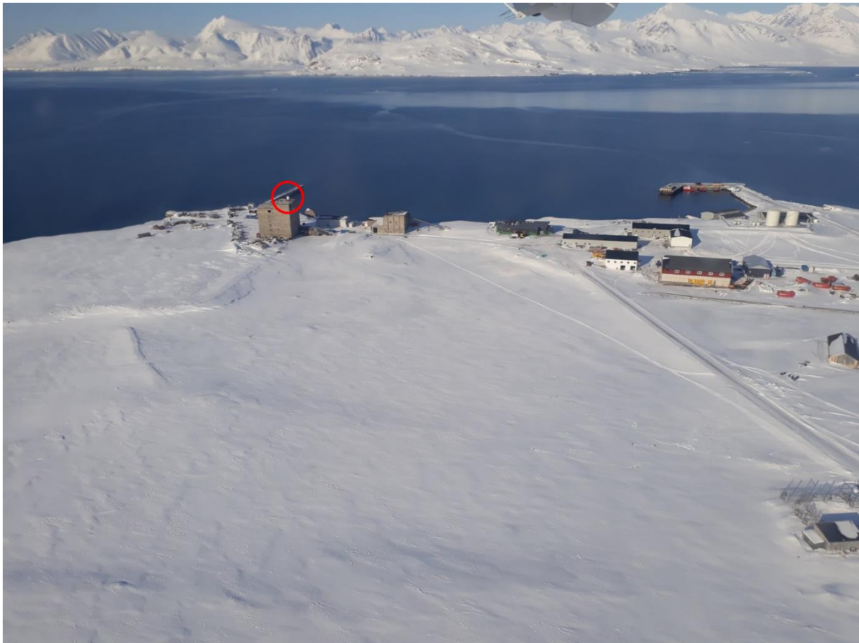
Figure 6: The GPRI's location (red circle) on the roof of an abandoned mining building in Ny-Ålesund (photo taken by Line Rouyet 26.04.2018).
