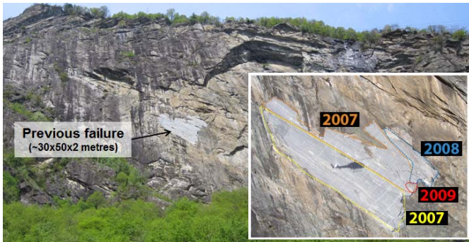
Figure 2 The rockwall at Soazza showing sites of previous block failure.
