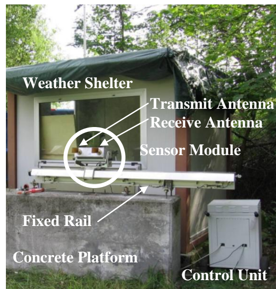
Figure 2.7. IBIS-L system at the Tessina landslide site (modified from Ingegneria Dei Sistem Online Brochure, 2007).
