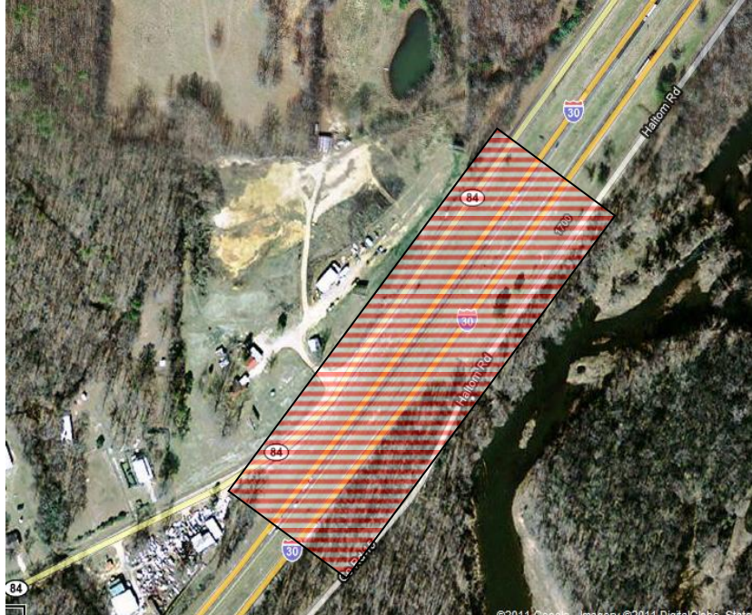
Figure 3.14. Location of project site located at Log Mile 95.7 on Interstate 30 near Malvern, Arkansas. Anticipated slide area shaded in red (Google Maps, 2011).
