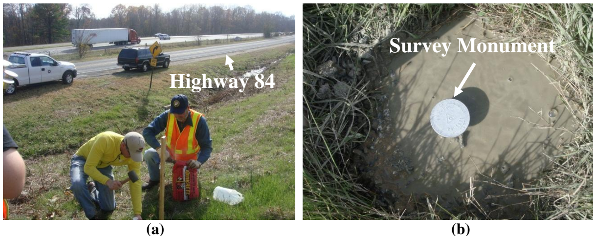
Figure 4.5. a) Installation of survey monument in the ground by UofA and AHTD personnel, and b) survey monument installed in the ground using Quickcrete®.
